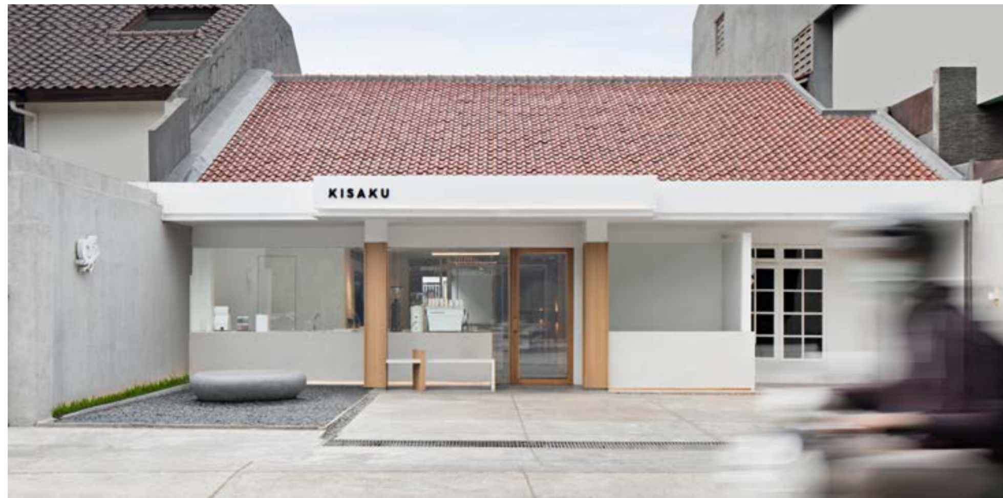
Shop front that preserves the existing house facade
